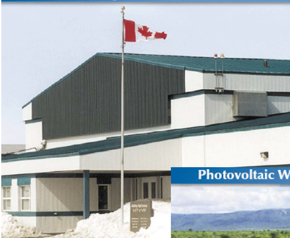
RETSCREEN® INTERNATIONAL Solarwall® on High School in Northern Canada
