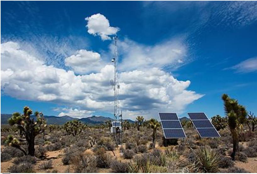
Fig. 1 Typical environmental sensor deployment with science, support, and communication systems. Photo 2013 Scotty Strachan, NevCAN Sheep Range Blackbrush station
